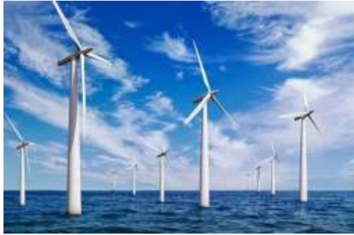
Offshore Wind Energy Farms
