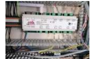
Concentrator (centralisation of data)
